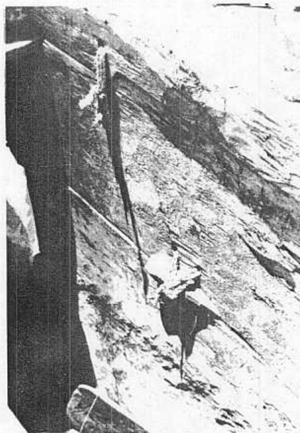
11. Method of lashing plank sides.
