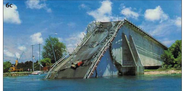
Fig 5. (left) Key features of original structural design and alterations made during remedial works Fig 6. (above & right) Photos showing the bridge after the collapse 22 (a) the whole span viewed from the Babelthuap side (b) Koror side (West) (c) Babelthuap side (East) (photo: © William E. Perryclear)
