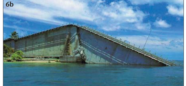
Fig 5. (left) Key features of original structural design and alterations made during remedial works Fig 6. (above & right) Photos showing the bridge after the collapse 22 (a) the whole span viewed from the Babelthuap side (b) Koror side (West) (c) Babelthuap side (East) (photo: © William E. Perryclear)
